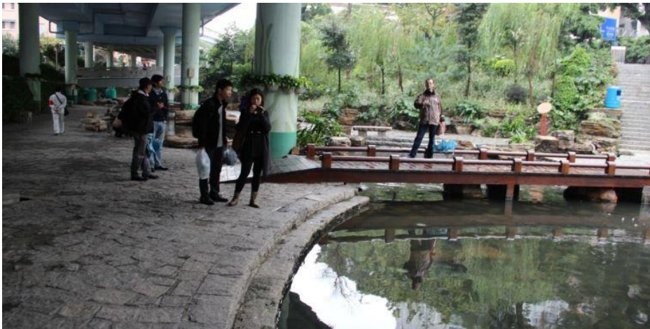
After the restoration of the canal; Photo credit: Lloyd Wright/ADB.
